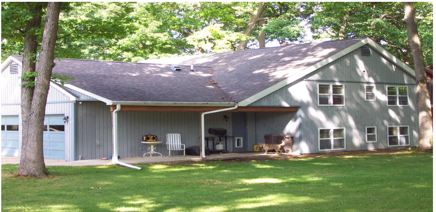
Rear view showing missing down spout extension.
