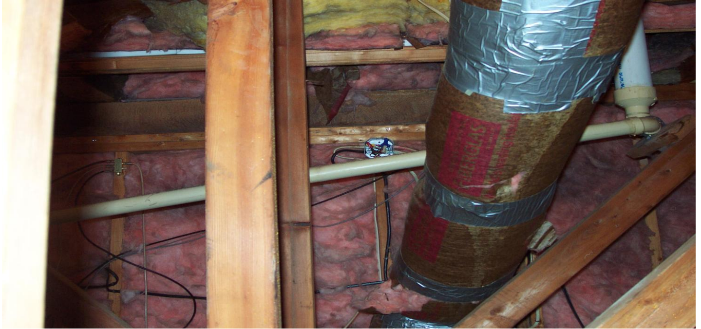
This electrical box in attic needs of cover. As seen from garage attic access.
